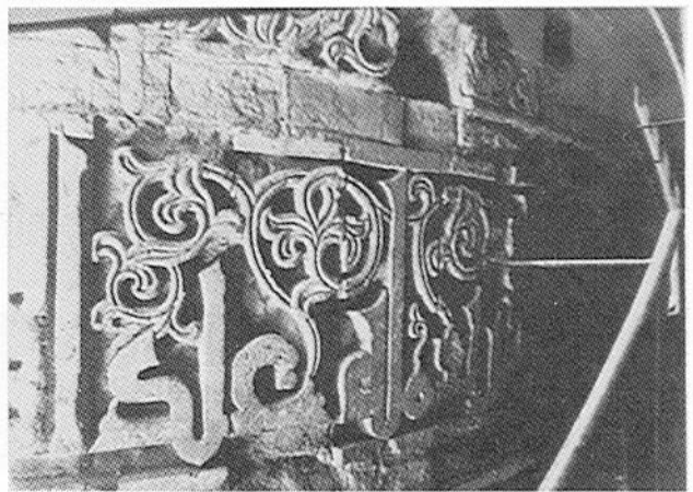
Pl. 49. Detail of the inner southwestern minaret of the mosque of al-Ḥākim (Creswell).
