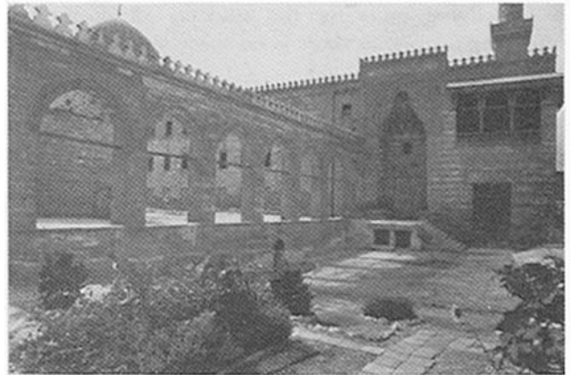
Pl. 98. The northern entrance of the khanqāh of Sultan Faraj Ibn Barqūq with a sabīl-kuttāb to its right.
