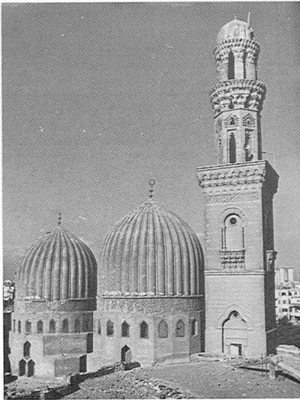
Pl. 72. The double mausoleum of the amirs Sanjar and Salār at the madrasa-khanqāh of Amir Sanjar.
