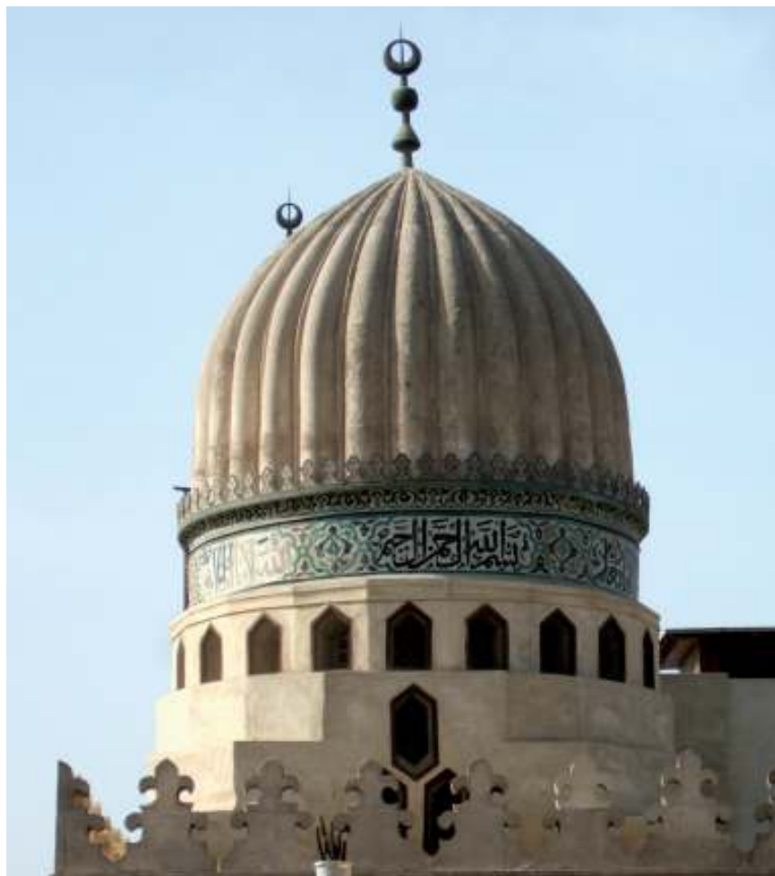
Figure 3: The mausoleum dome of Emir Aslam al-Silahdar (1344–45) with tile mosaics in the drum.
