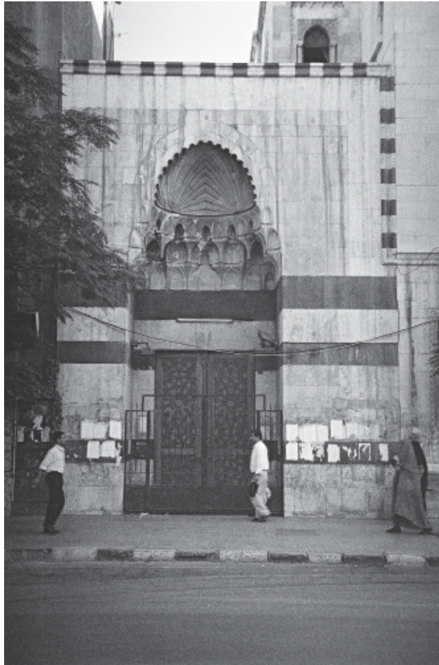
Figure 4: Damascus, mosque of Tankiz, west portal.
