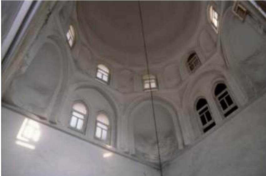
Figure 6: Damascus, mausoleum of Tankiz, interior of dome.
