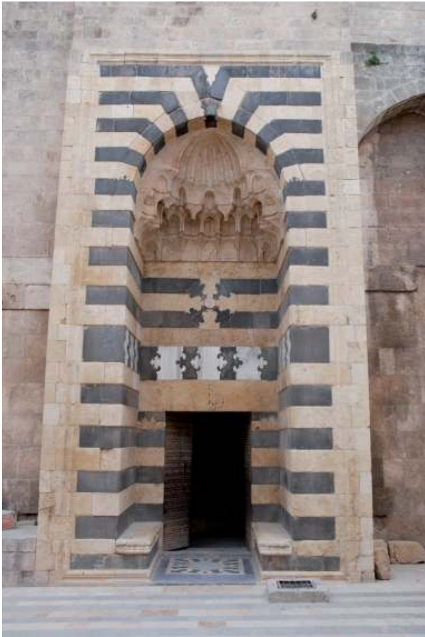
Figure 11: Northern portal of the Throne Hall.
