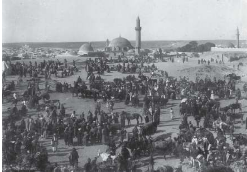
Figure 15: View from the Aleppo Citadel to the former Friday Market.
