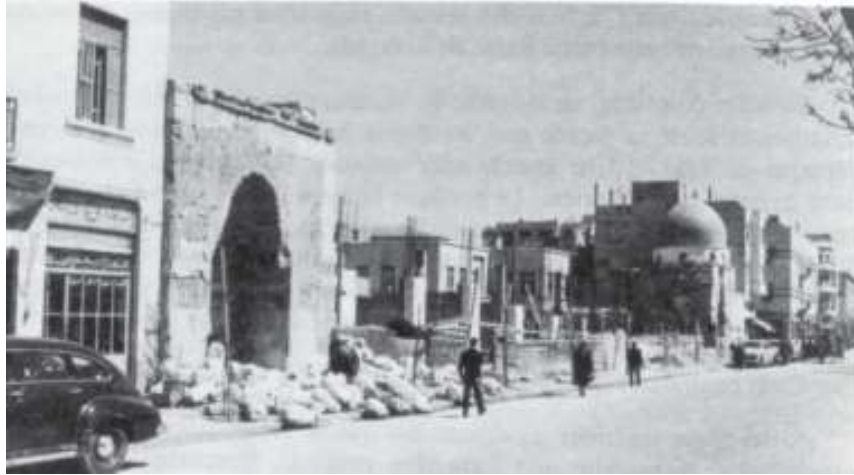
Figure 1: Damascus, mosque of Tankiz during demolition.
