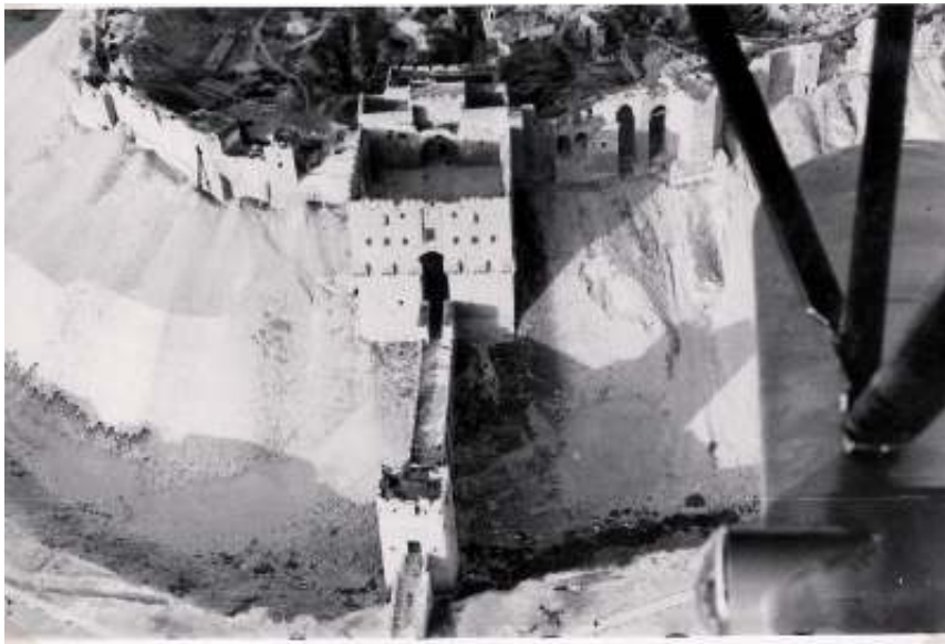
Figure 3: The Throne Hall without roof before restorations, 1935–36.
